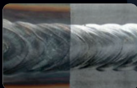
cleaning of welding seams
